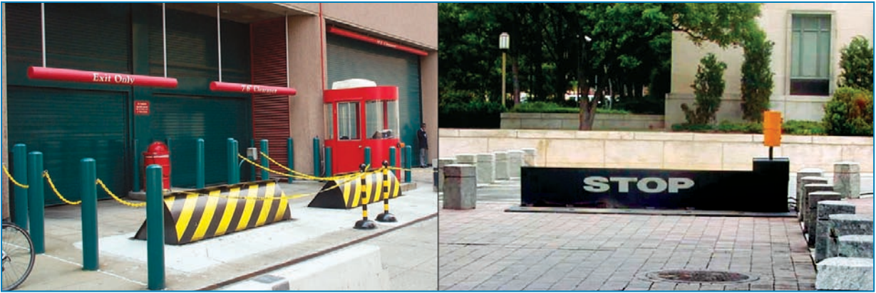
Figure 4-41: Rotating wedge installation with typical manufacturer’s jazz pattern (left), rotating plate barrier with stop sign in an elegant font combined with well-designed fixed low bollards (right).
