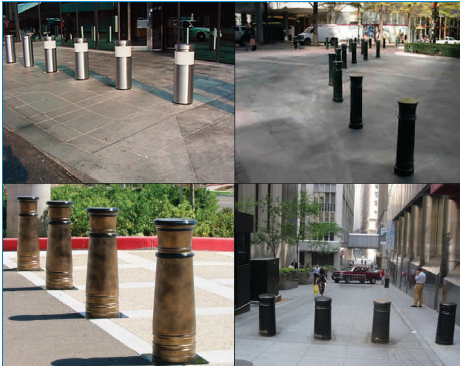
Figure 4-18: Decorative bollards with high-performance ratings.
