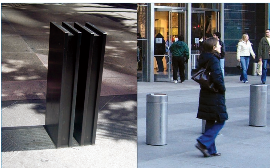
Figure 4-19: Custom-designed steel bollards that match the design of their buildings
