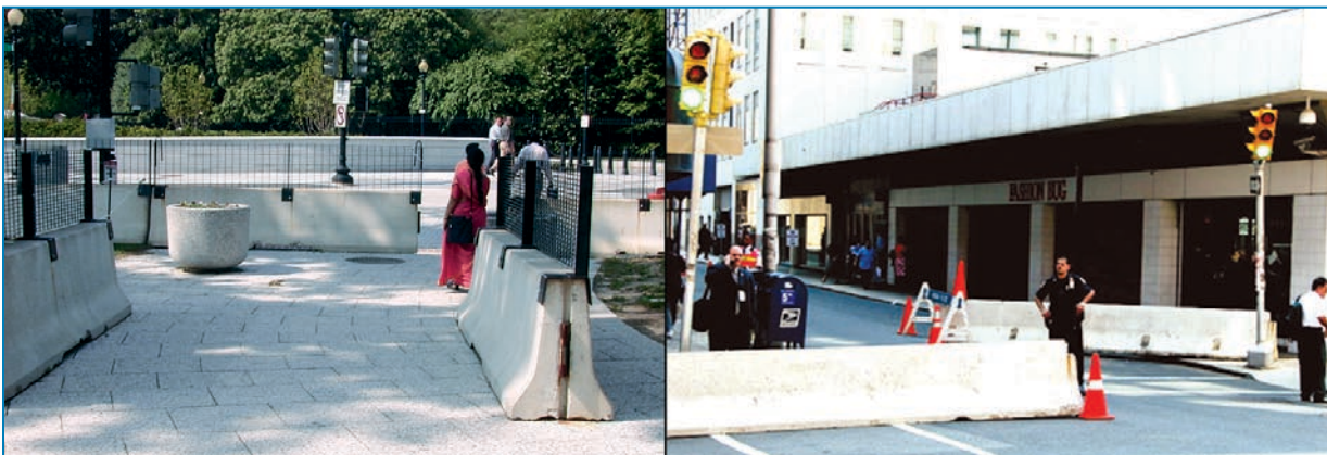
Figure 4-29: Jersey barriers: pedestrian disruption at the White House (left) and on a D.C. Street (right).
