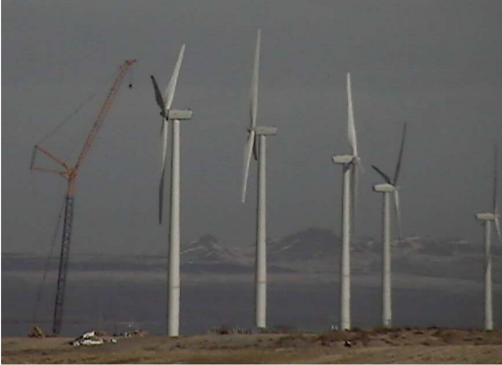
Figure 9: Construction Photo of Fossil Gulch Wind Farm with 300 ton crane
