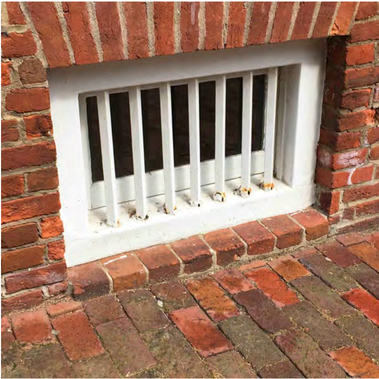
Basement window casing nearly 4" wide
