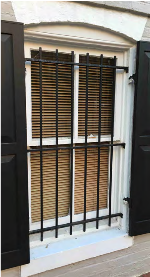
Note flat wood arches and modified bullnose brickmould
