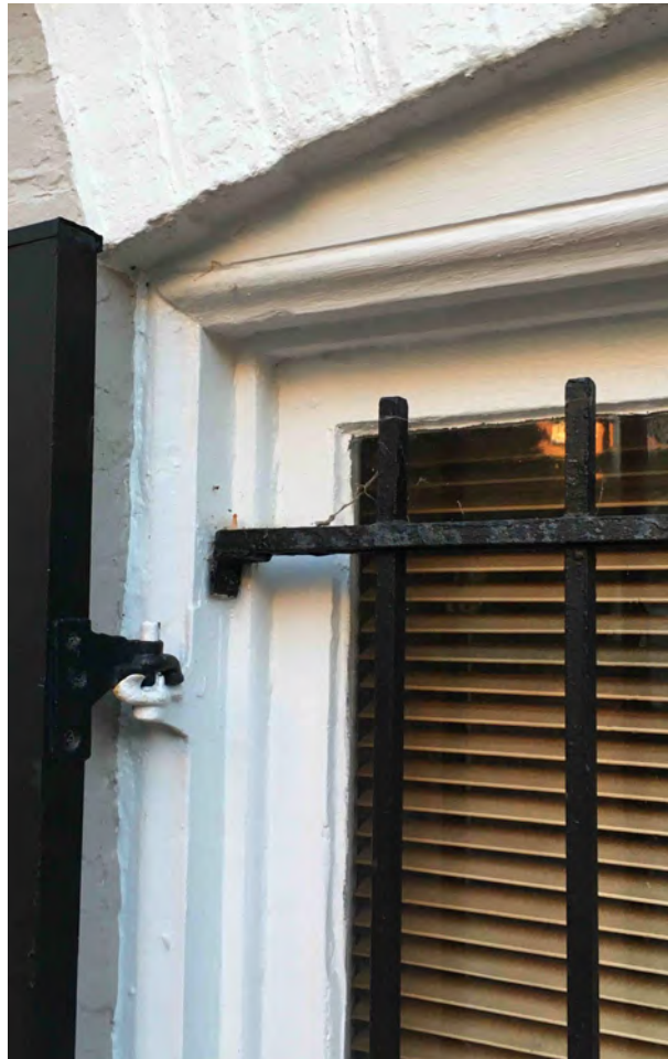
Note flat wood arches and modified bullnose brickmould
