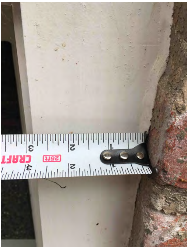
Existing Basement window casing – 2-3/4" wide
