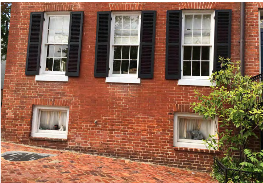
Basement window casing nearly 4" wide / Brickmould on first and second floors 1-3/4" wide
