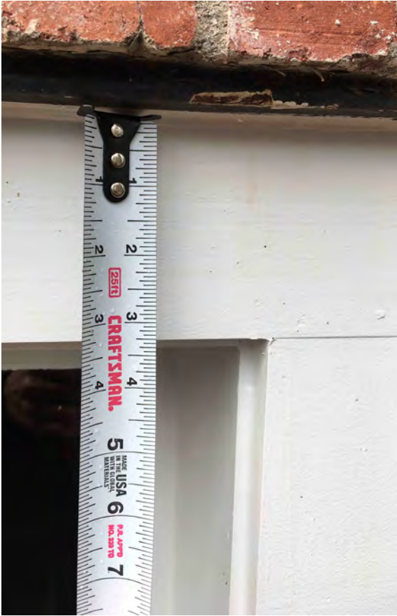
Existing Basement window casing – 3-1/2" wide
