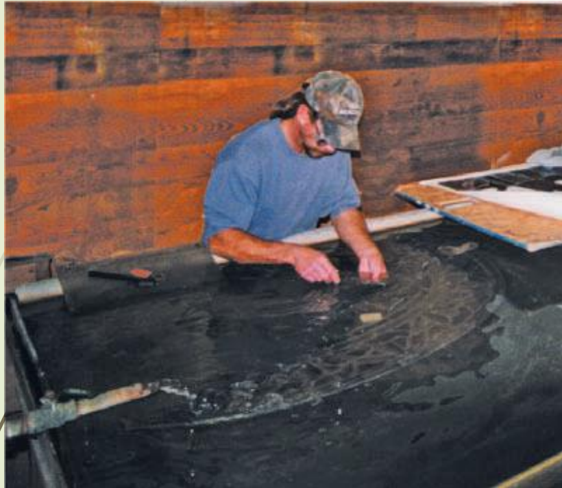
Restoration technician carefully disassembles a window under water in a specially designed lead reclamation tank
