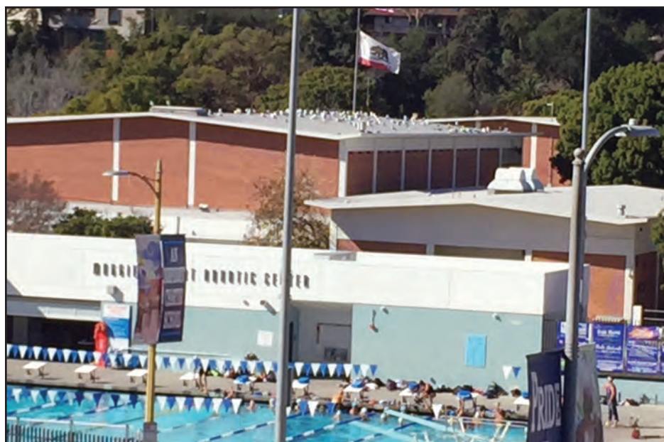
Instead of seagulls on the roofs of PaliHi, administrators would like to see solar panels.
