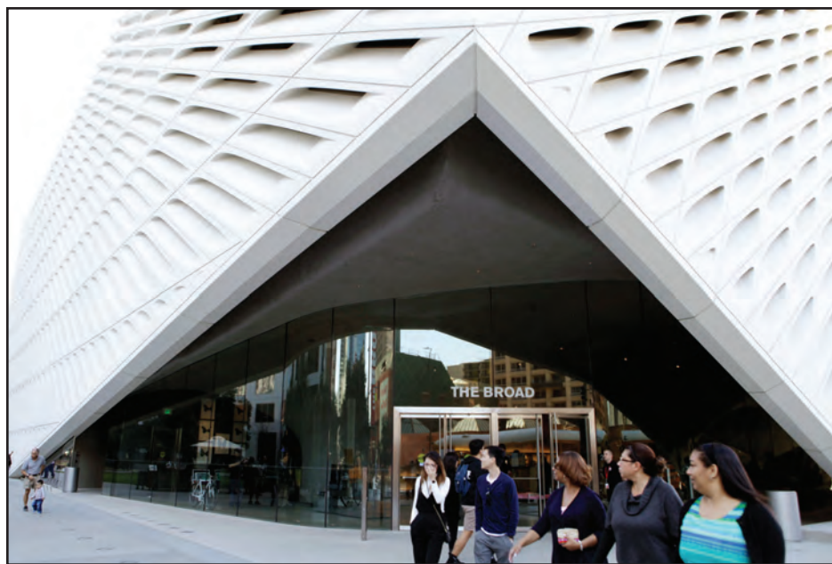
The Broad, built by philanthropists Eli and Edythe Broad on Grand Avenue, features the veil-and-vault design by Diller Scofidio + Renfro.
