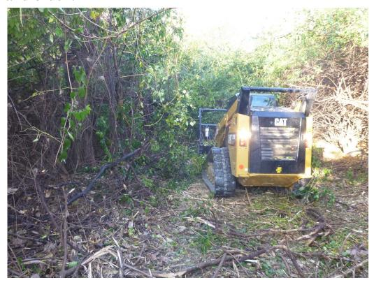
Photo is taken inside the OU1, near the reference area 23, the view is facing west. The pathway is being cleared of debris and vegetation. The dust suppression method, if necessary, is to lightly wet the material to keep fugitive dust and visible emissions to a minimum in dry and high wind conditions. There were no visible dust emissions observed during cutting operations.
