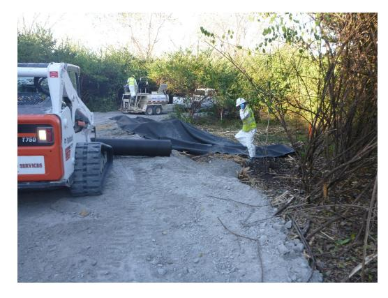
Photo is taken inside the OU1, near the reference area 23, the view is facing west. The pathway is being cleared of debris and vegetation by a forestry mower bobcat. The forestry mower is used to cut small trees and brush.
