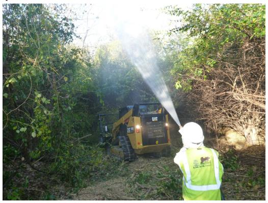
The view is facing southeast and shows what the forestry mower / cutter attachment on the bobcat looks like. The forestry mower is used to cut small trees and brush in preparation for grading a pathway through the site for the additional testing and characterization.
