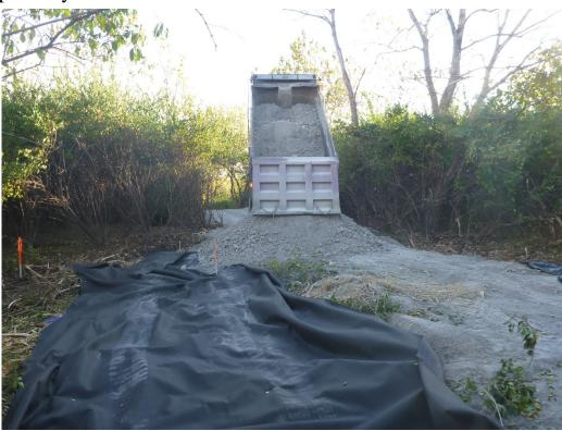
Photo is taken inside the OU1, near the reference area 23, the view is facing west. The pathway is being cleared of debris and vegetation. The photo shows roughly how the area is staked out, the underlayment padding/matting for the path and the crushed gravel used in paving the pathway. The dust suppression method, if necessary, is to lightly wet the material to keep fugitive dust and visible emissions to a minimum in dry and high wind conditions.
