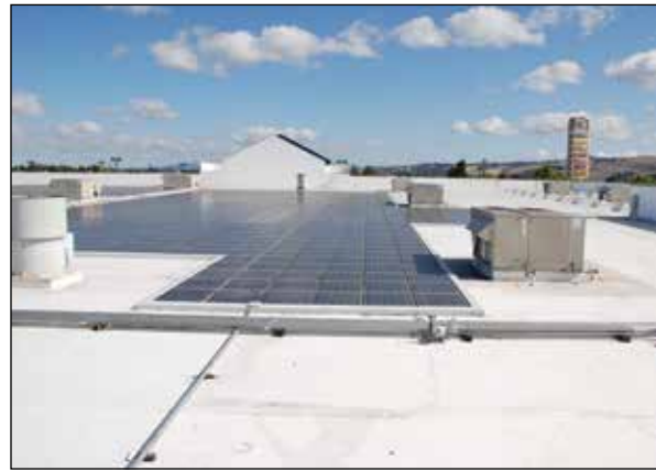
Photo 1.3 • Commercial PV array mounted horizontally with some shading.
