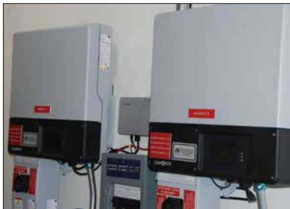
Photo 1.16 • Transformerless (non-isolated) inverters, typically used on most recent residential and small commercial PV systems. Courtesy of SMA Technologies AG.
