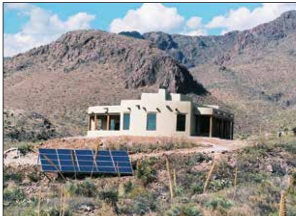
Photo 1.2 • 3.3 kW stand-alone, off-grid PV system.
