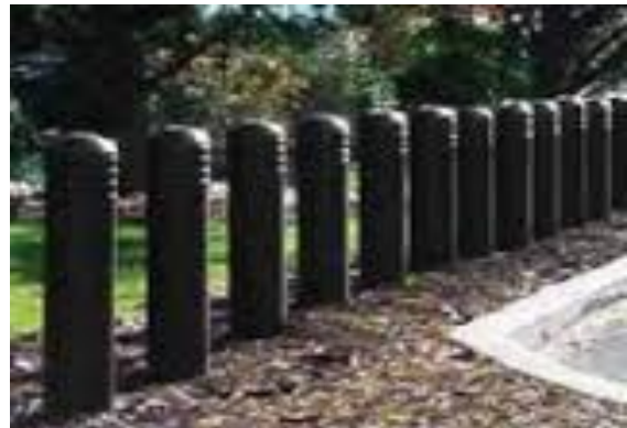
Figure 2. Passive Barrier (Illustrative Examples)
