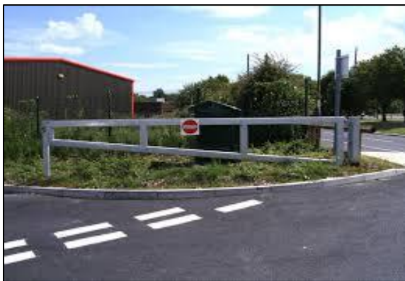
Figure 4. Manually Operated Active Barriers (Illustrative Examples)
