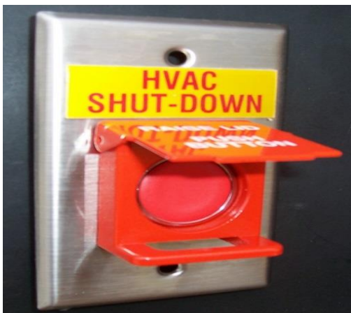
Figure 6. HVAC Emergency Shut-Down Switch Cover (Illustrative Examples)
