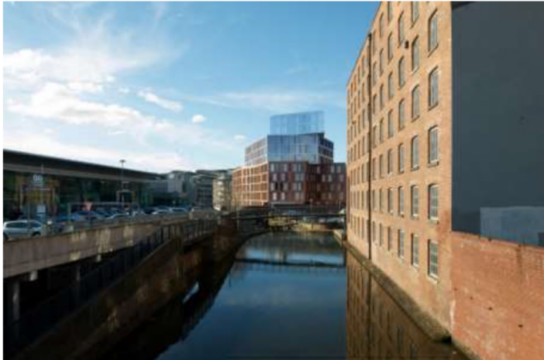
Tariff Street Key View: From Great Ancoats Street canal bridge crossing, looking south down the canal (source: 106021/FO/2014/C2)
