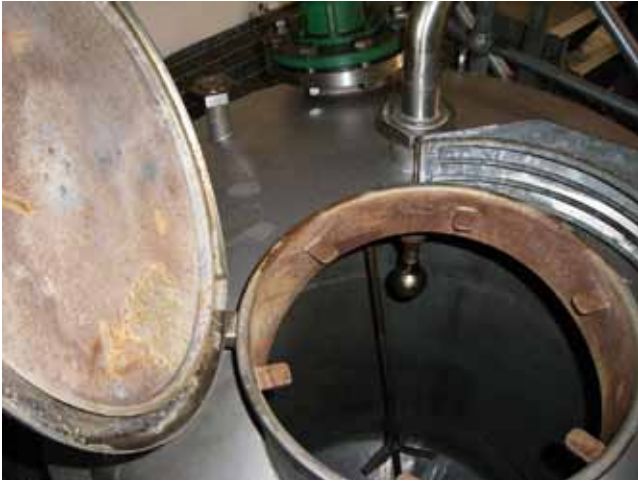
Surface rust – before and after removal using Avesta Cleaner 401.
