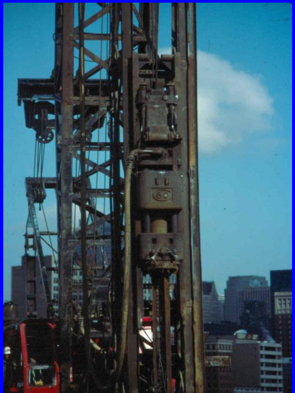
Differential Acting Air Hammer
