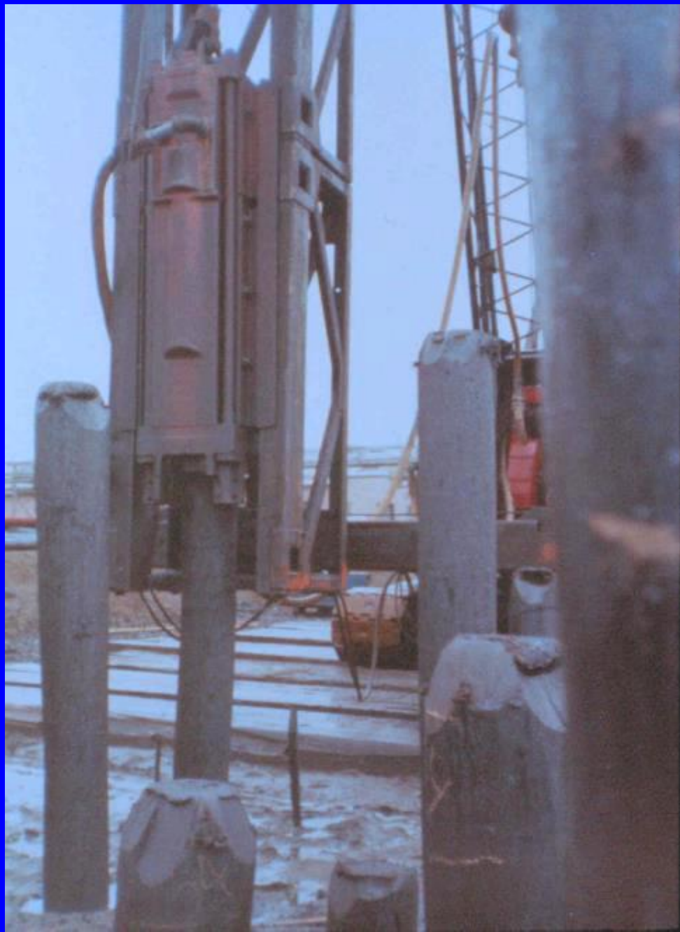
Double Acting Air Hammer
