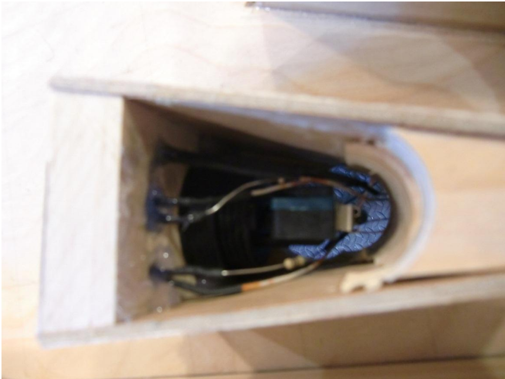
Installation of push-button and LED's near IR switch
