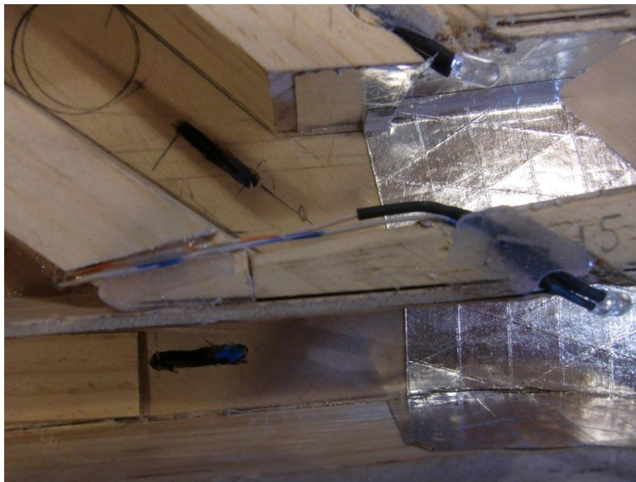
Floor switches an embedded LED's at mouth of channels.
