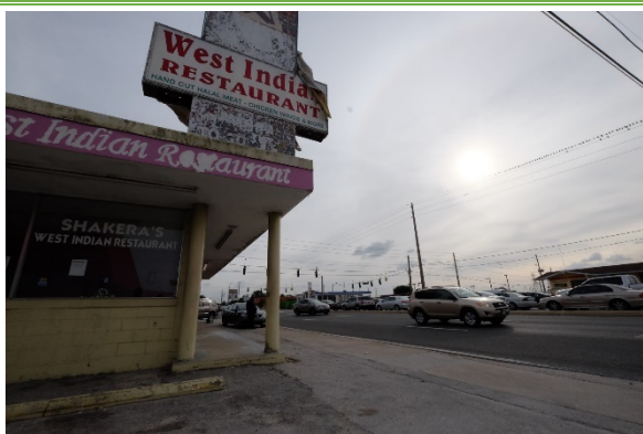
Image 2: Shows the state of degradation buildings are in and the quantity of utility lines
