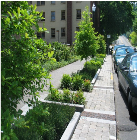
Image 6: Another example of maintenance and natural access control.
