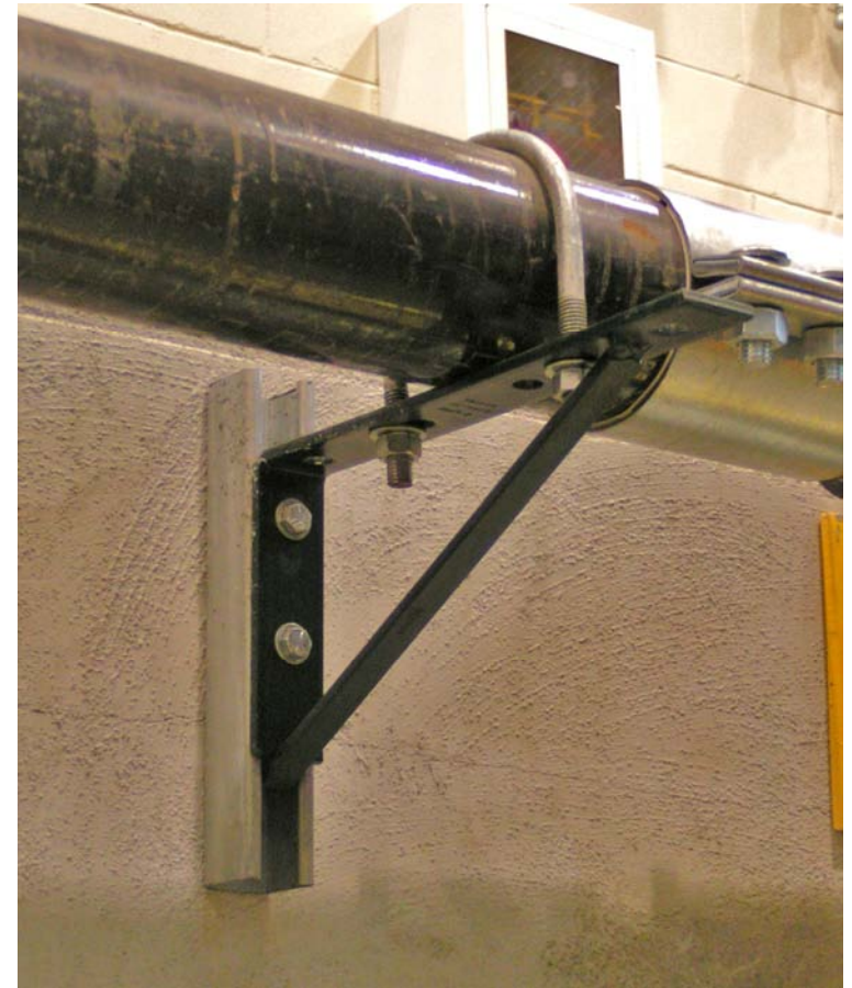
Schedule 40 steel pipe material shown with unistrut / fabricated wall support and U-bolt.
