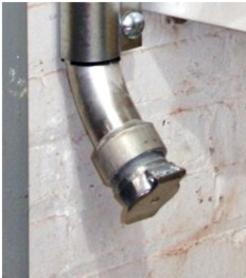
Inlet Valve has 2" NPTM thread and screws into the adaptor elbow
