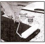
Roll thin coat of 520 or 520 BLV Adhesive to insulation.
