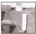
Insulate sides first. Apply thin, uniform coat of Armaflex 520 or 520 BLV Adhesive.
