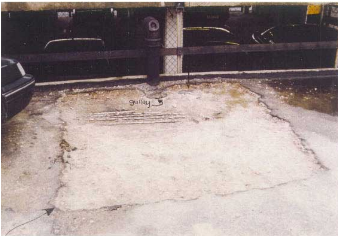
Figure 6.1 - 1 CDM photo [H126] of initial cutting out at J2, January 1996.
