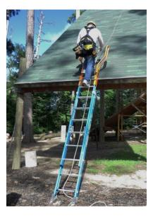
Lateral Slippage is the second most common cause of ladder related failure. It can take place with as little as 9 lbs of pressure during the climber's lateral transition from ladder to roof or roof to ladder. Both kick-out and lateral slippage greatly reduced with can be the implementation of ladder stabilizing accessories.
