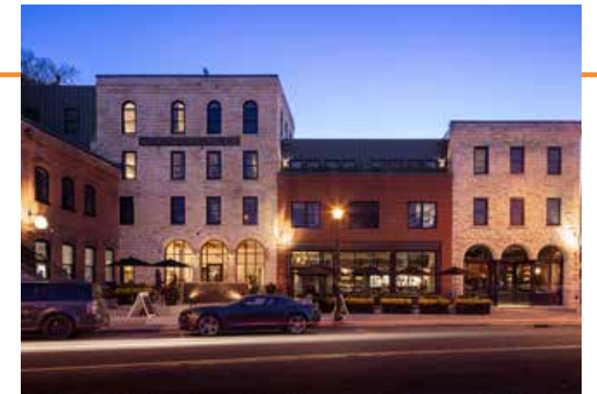
Stakeholders: Braun Intertec, Emanuelson-Podus, Erickson Civil, ESG Architecture & Design, Express Fire Protection Services, Innovative Structural Solutions, Laketown Electric Corp, Northern Mechanical Contractors, Stillwater Heritage Preservation Commission, Zeman Construction
