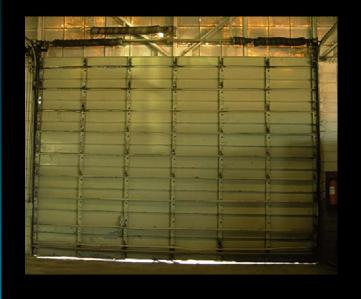
The torsional spring located at the top of the garage door winds up as the door is lowered. When the door is raised, the potential energy stored in the spring is transferred into the gravitational potential energy of the door's weight, thereby making it easy to open.
