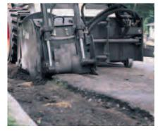
The **oscillation** of the planer provides optimum surface tracking and isolating the planer from loader movements caused by uneven terrain. Adjustable depth skis allow tapering of cut, such as when matching two uneven pavement surfaces or removing a curb ridge.
