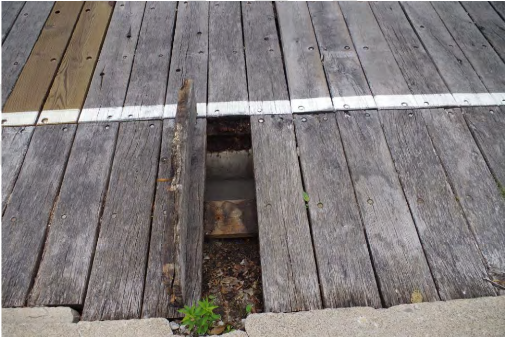
Figure B-2: Top View of Gutter at North Trail
