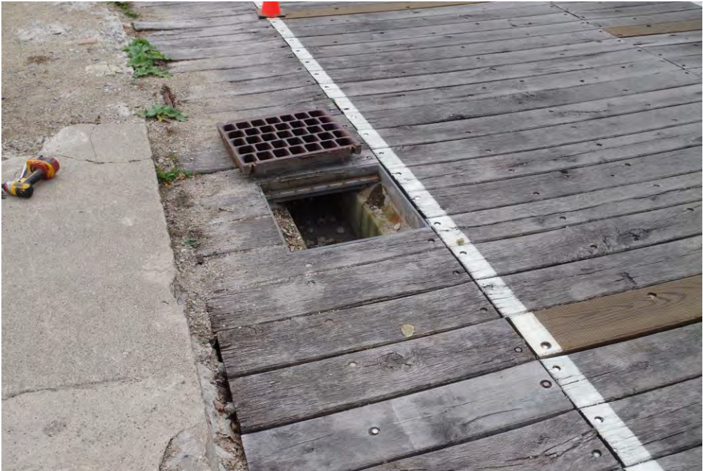
Figure B-1: Drainage Grate on North Trail
