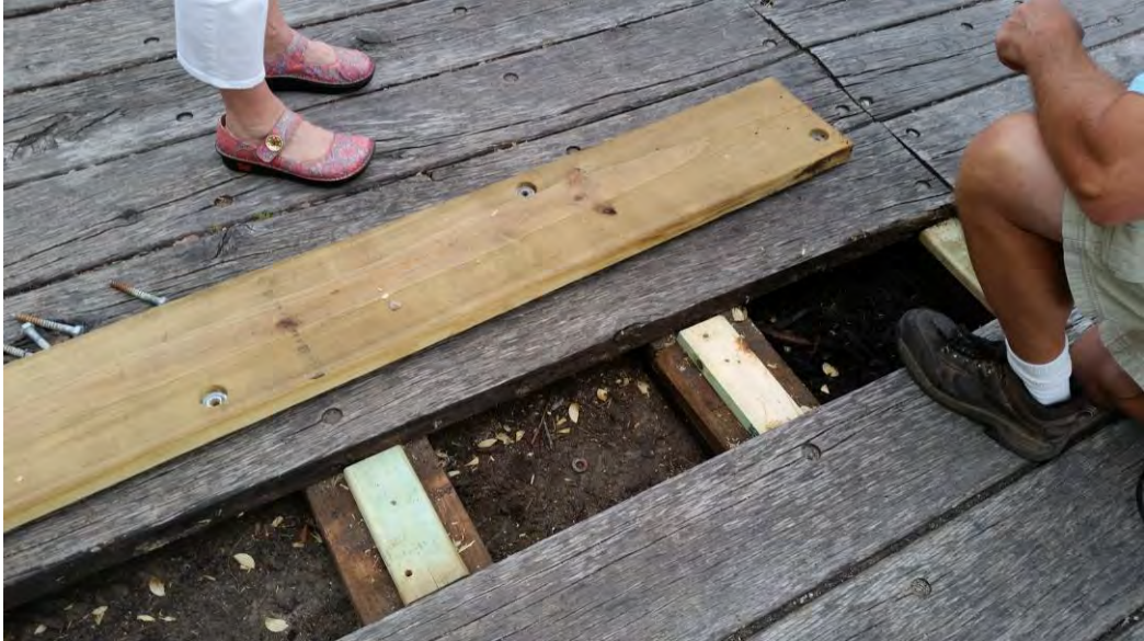
Figure B-5: Replacement Plank at South Trail (Concrete Base)
