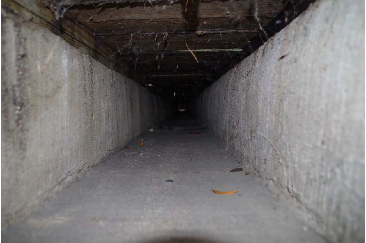
Figure 14: Concrete Gutter System on North End of Trail
