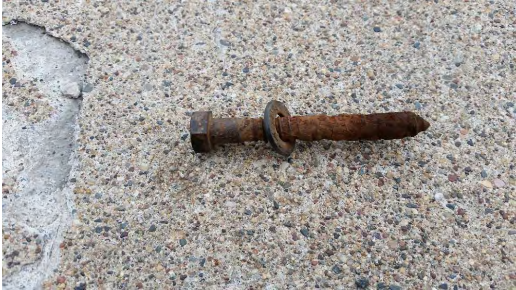
Figure B-6: Corroded Bolt with Thread Loss
