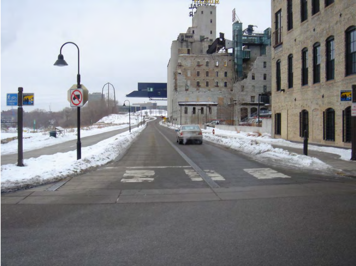
Figure B-12: Plank Road in winter before Road was Rebuilt (Circa 2010)
