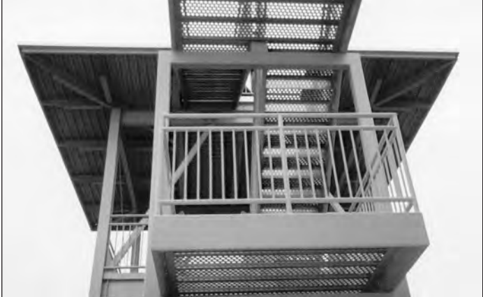
PERF-O GRIP® Plank Grating makes a unique non-slip stairway and platform for this observation tower.
