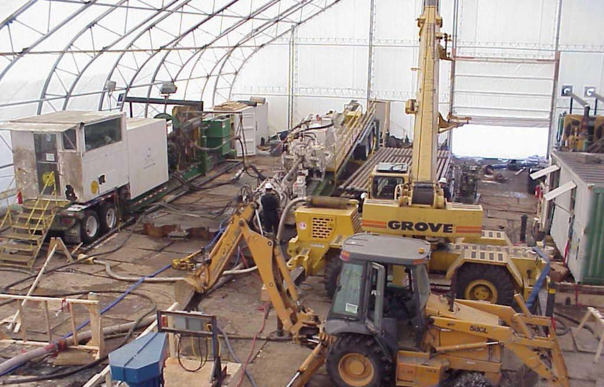
Drill Entry Winter Enclosure
