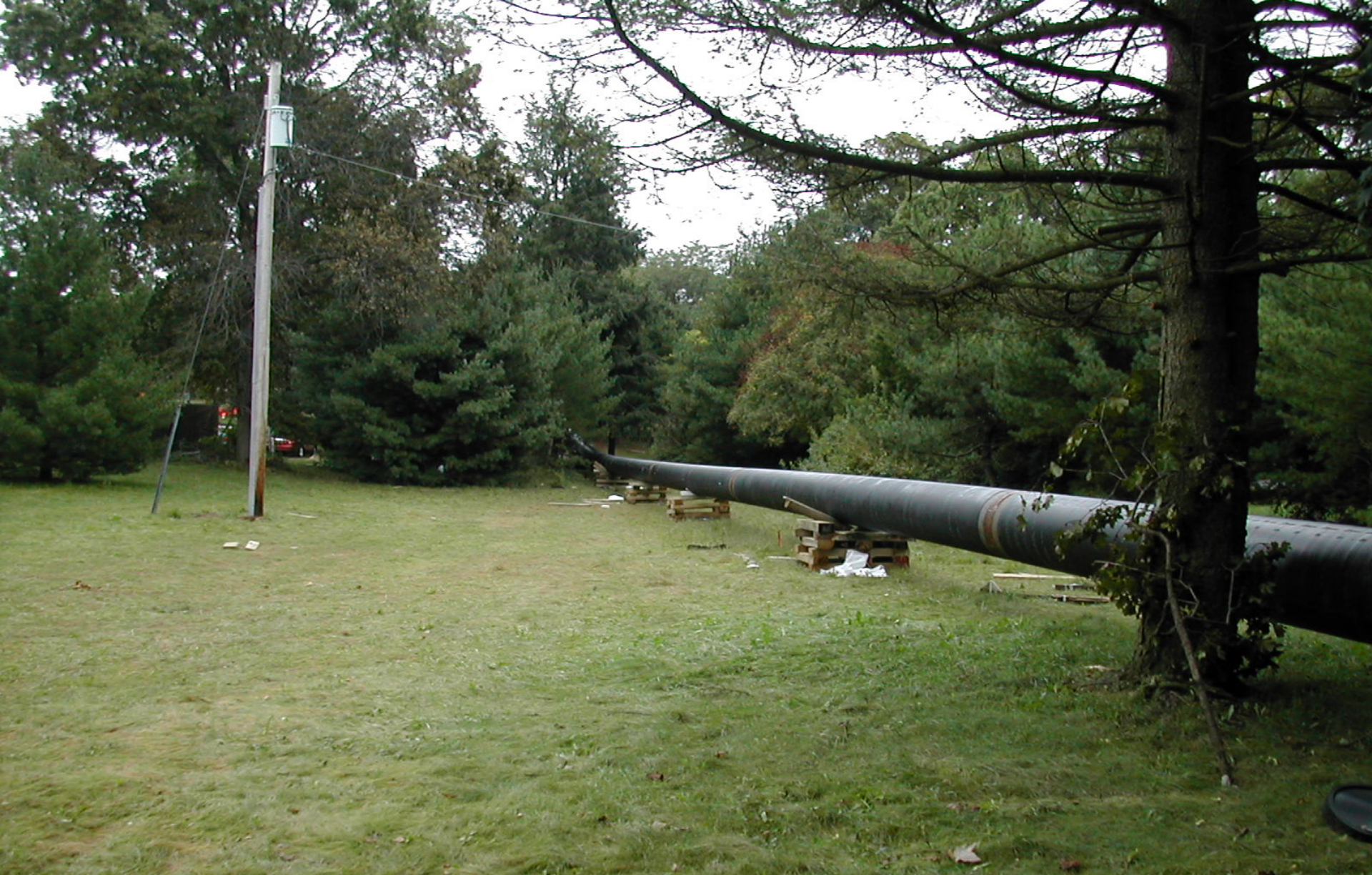
Drill Exit Pull Section
