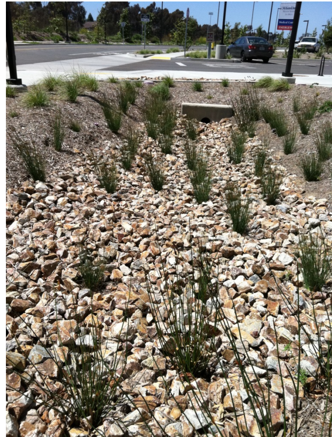
Parking lot bioretention
