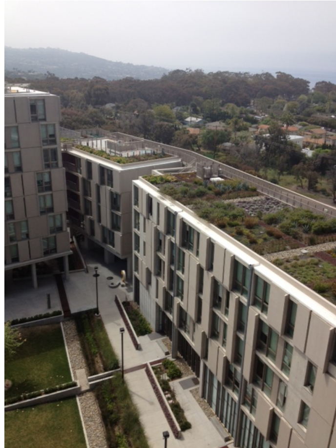
Green roof on Keeling Apartments at UC San Diego
