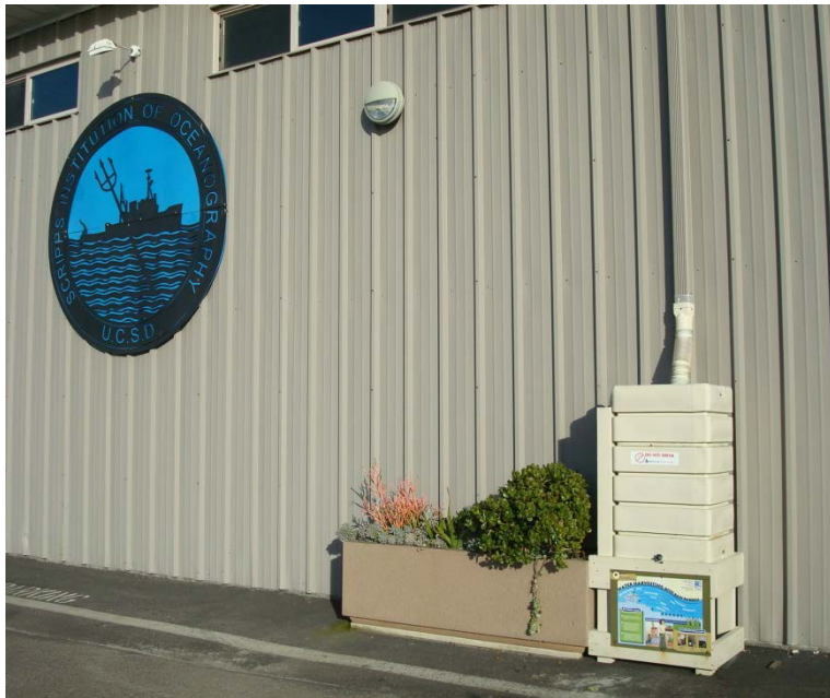
Rain barrel and planter box system at Scripps Institution of Oceanography
