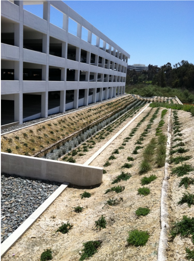
Parking structure bioretention
