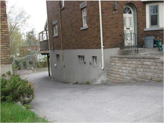
Figure 2: View looking east at 923 Bronson, slope is visible.
