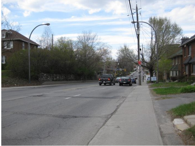
Figure 7: View looking north on Bronson. Shows west side of the street.
