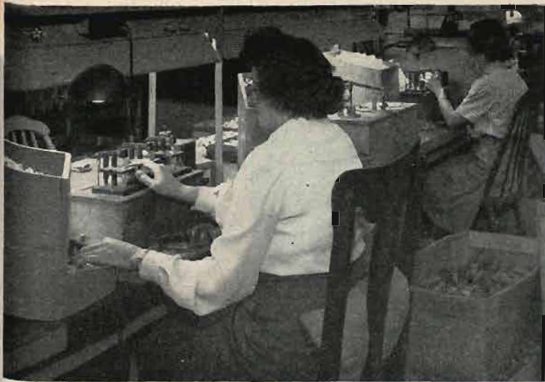
CAREFULLY CONTROLLED PROCESS, workers here are fusing together the plastic bodies.
