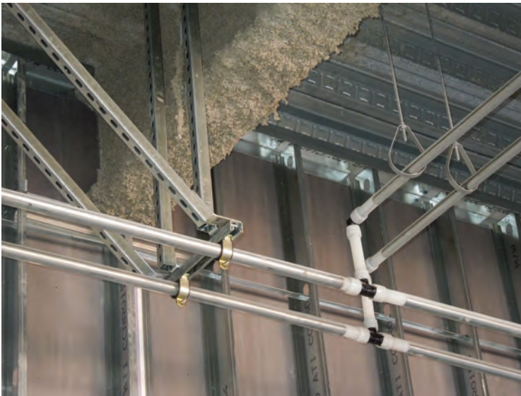
Figure 5-1: Uponor PEX-a Pipe Support
