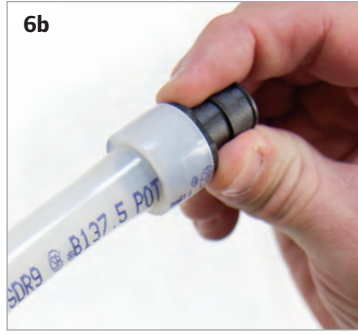
Insert ProPEX Fitting into 1/2" Uponor PEX Piping.
