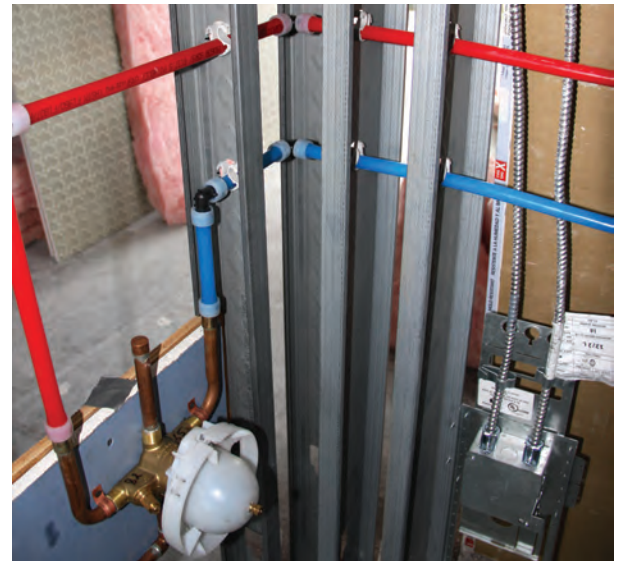
Figure 5-2: In-wall Piping
