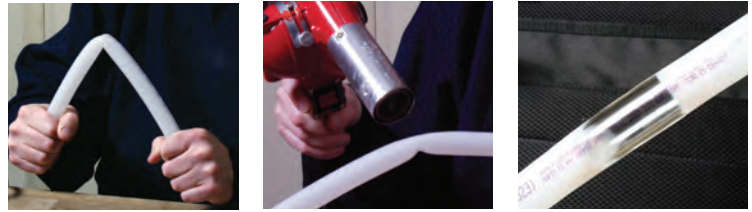
Figure 6-2: Reforming Kinked Piping
