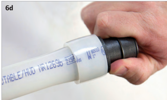
Insert ProPEX Fitting into 1" Uponor PEX Piping.
