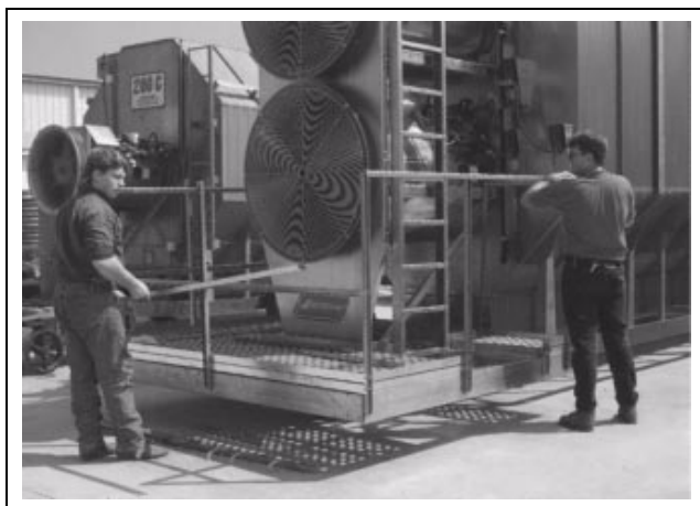
Figure 2X Installing Front and Side Upper Guard Rails
