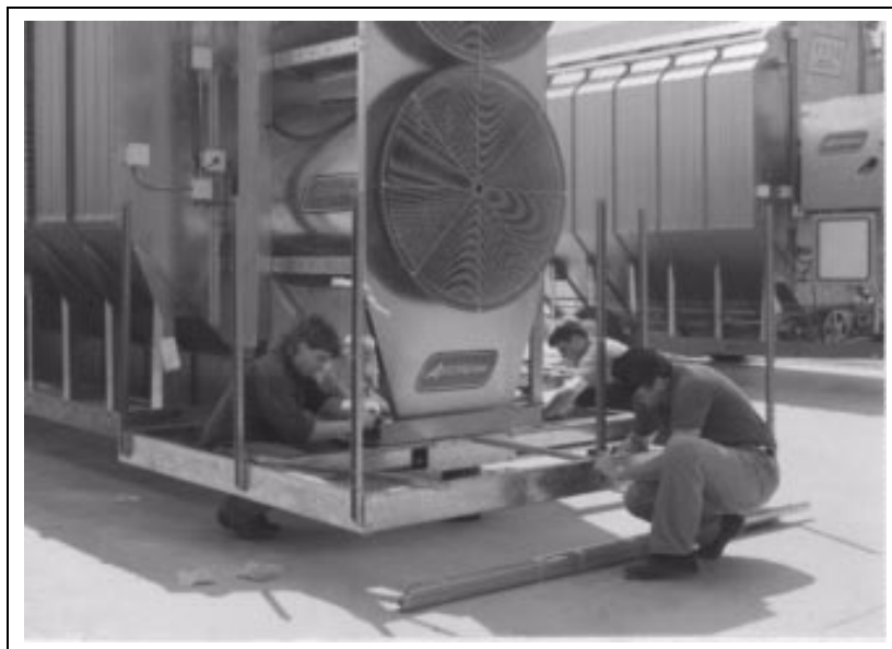
Figure 2P Install Remaining Support Channels
