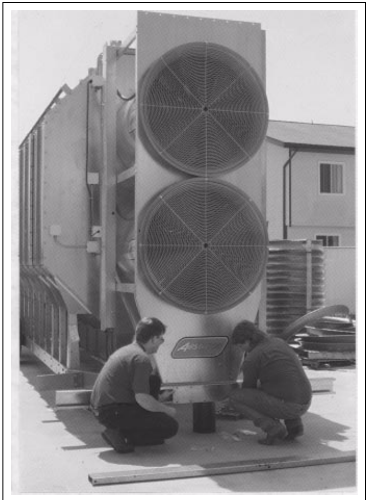
Figure 2C Mounting the Main Support Channel
