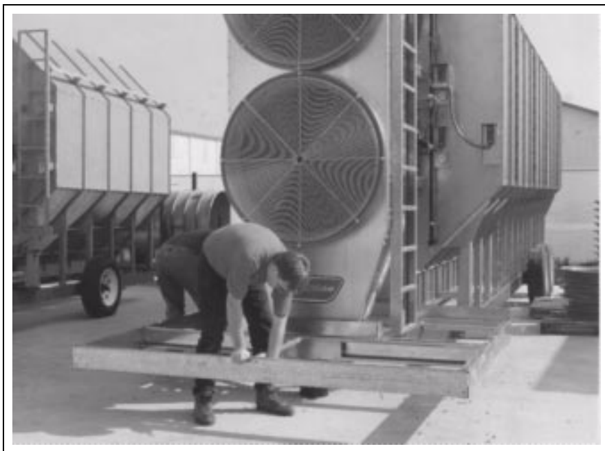
Figure 2J Center Floor Support Placement
