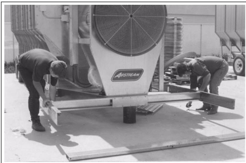
Figure 2E Attaching Side Channels
