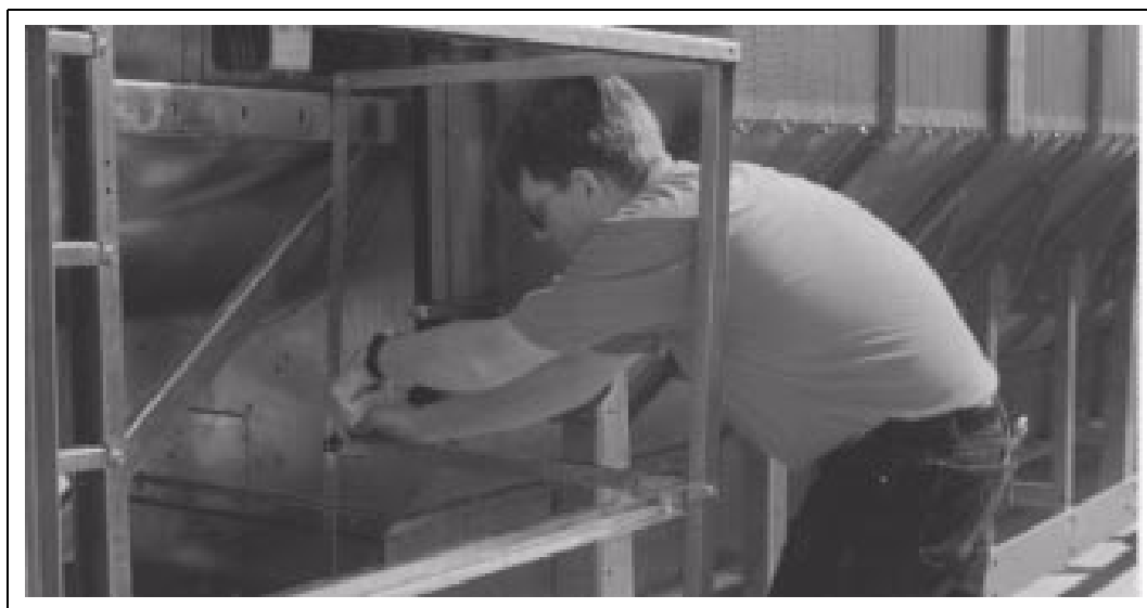
Figure 2Z Installing Lower Rear Guard Rail
