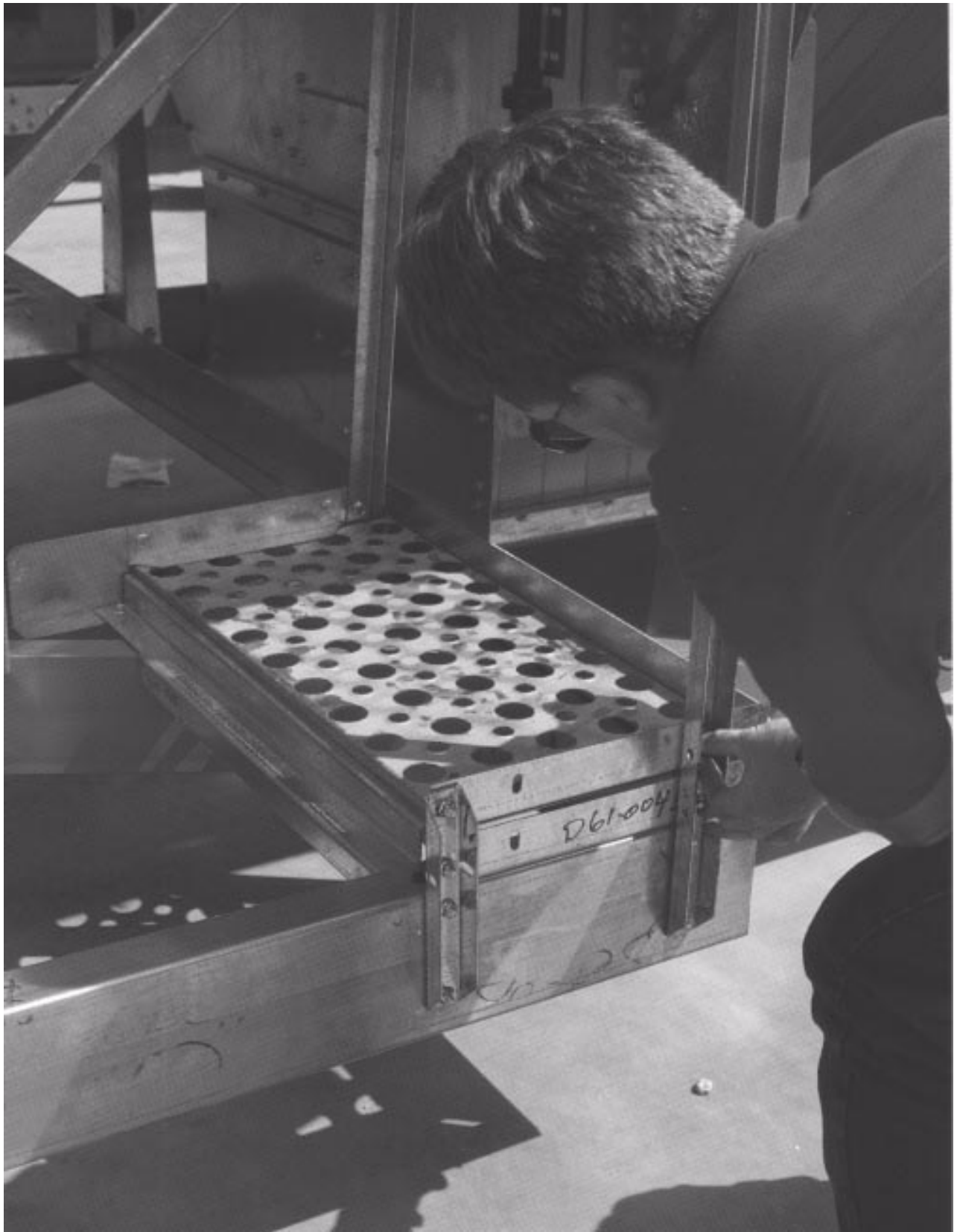
Figure 2W Installation of the short wide floor panel, left hand outer rear toe boards and hinge channel.
