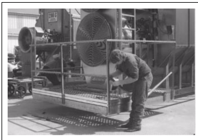
Figure 2Y Installing Lower Side Guard Rails
