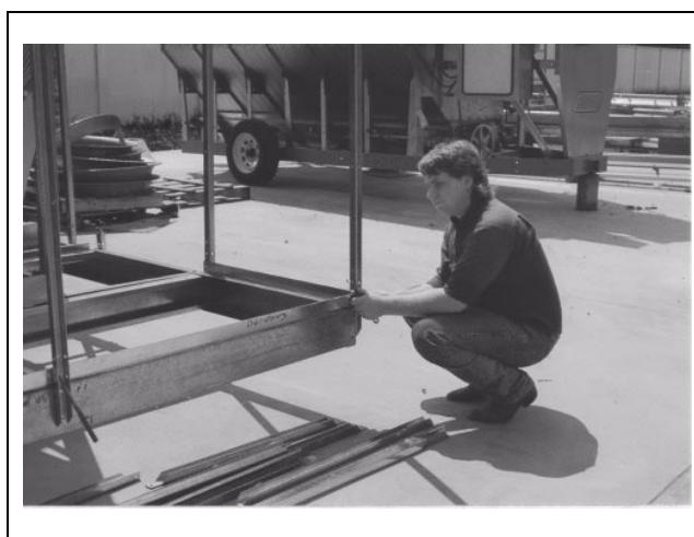
Figure 2R Connecting Left Hand Front Toe Board to Guard Rail Support Channel
