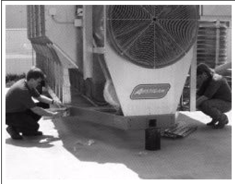
Figure 2B Connecting Rear Anchor Channels
