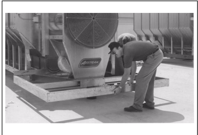
Figure 2I Attaching Front Channel
