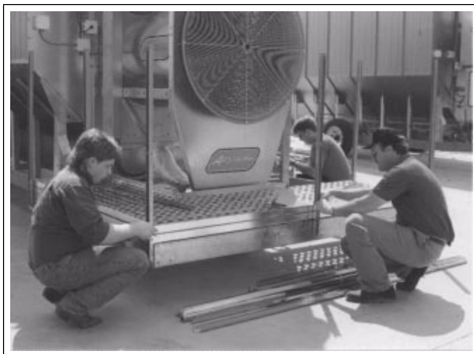
Figure 2V Installing the Remaining Toe Boards
