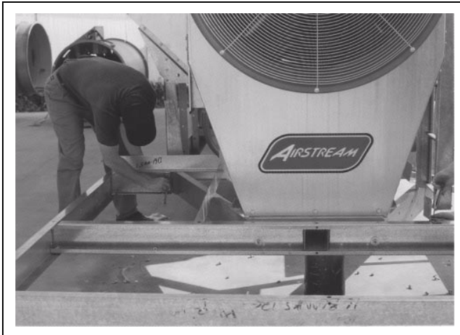
Figure 2G Tighten the Rear Frame Tie Angle to the Side Frame
