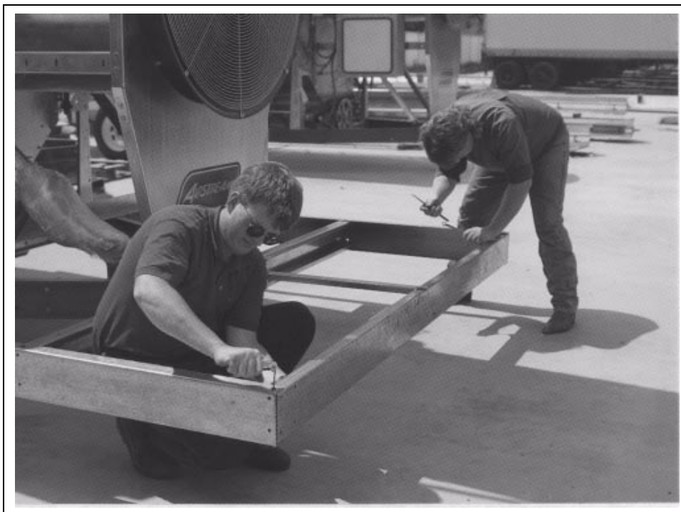
Figure 2K Check for Squareness and Tighten Bolts
