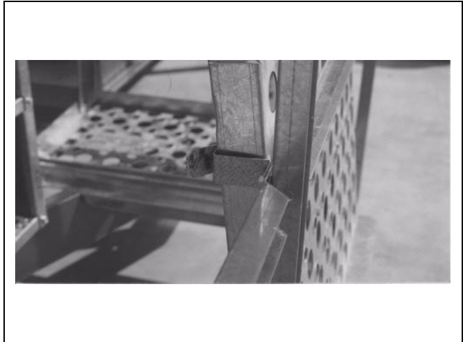
Figure 2AC Close-Up of Access Door Clip on Guard Rail
