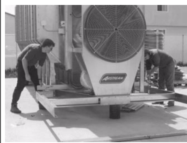
Figure 2F Placing Rear Tie Angle on Platform
