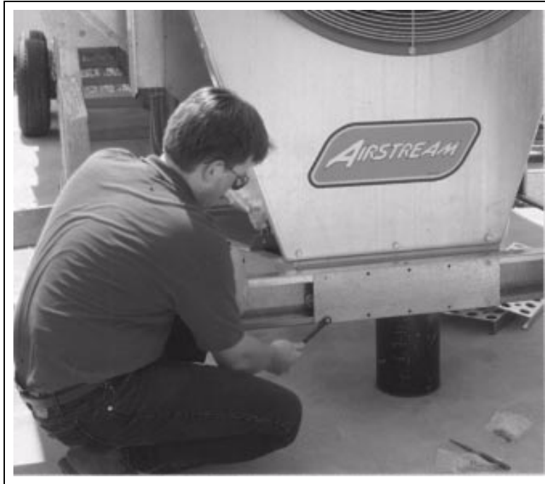
Figure 2D Bolting Reinforcement Plate to Main Support Channel
