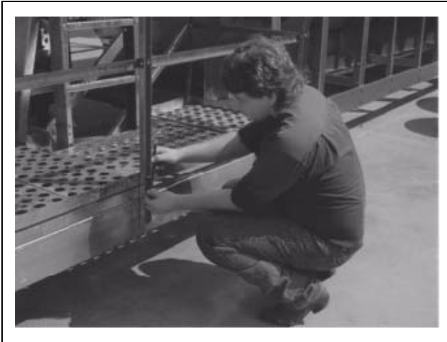
Figure 2AA Installing Access Door
