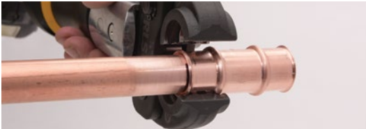
1. Insert the tube in the fitting
