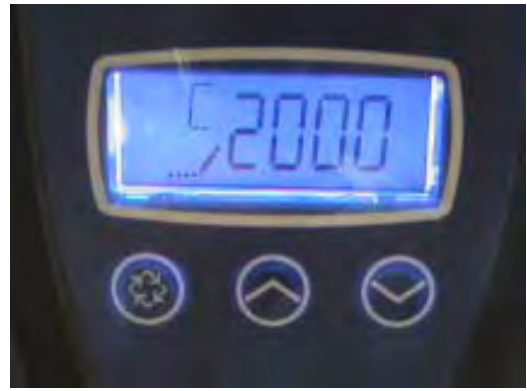
Fig 2. Ecosmarte® Control Valve is displaying the 2000 gallon backwash interval. (Low volume user). Typical settings for granular activated carbon tanks are 1000 gallons for low volume users, 2000 gallons for average and 3000 gallons per months for large families or when outdoor water is used. (On well water GAC valves use pins 6 and 12)
