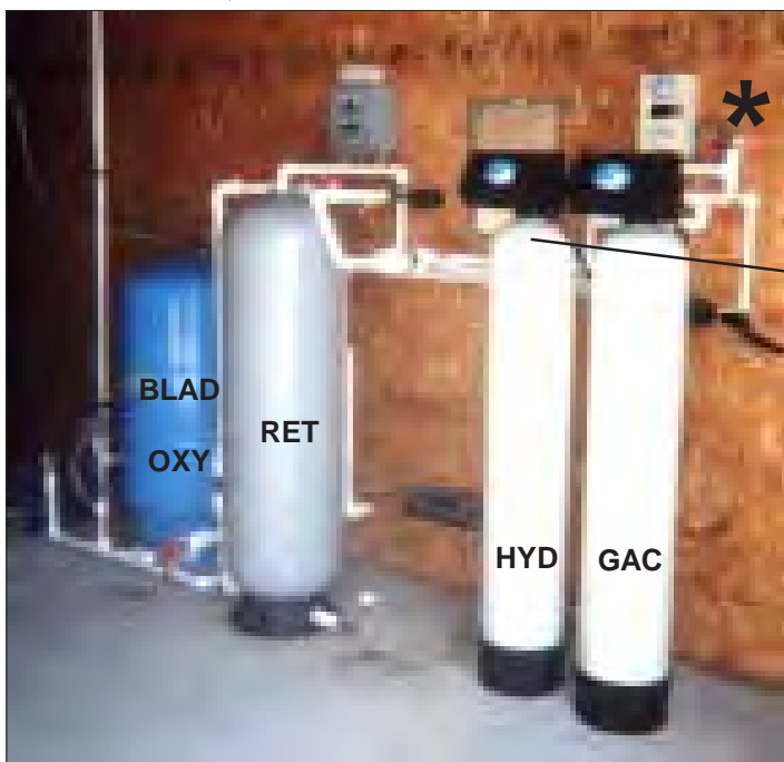
Fig. 3: Left to Right: Wellmate, Well, Bladder Tank, OXY Chamber, Hydroxite Tank with Valve Sensor, ECOsmarte® Valves, Carbon Tank, Cu Chamber (behind GAC), (Water to Home.)
