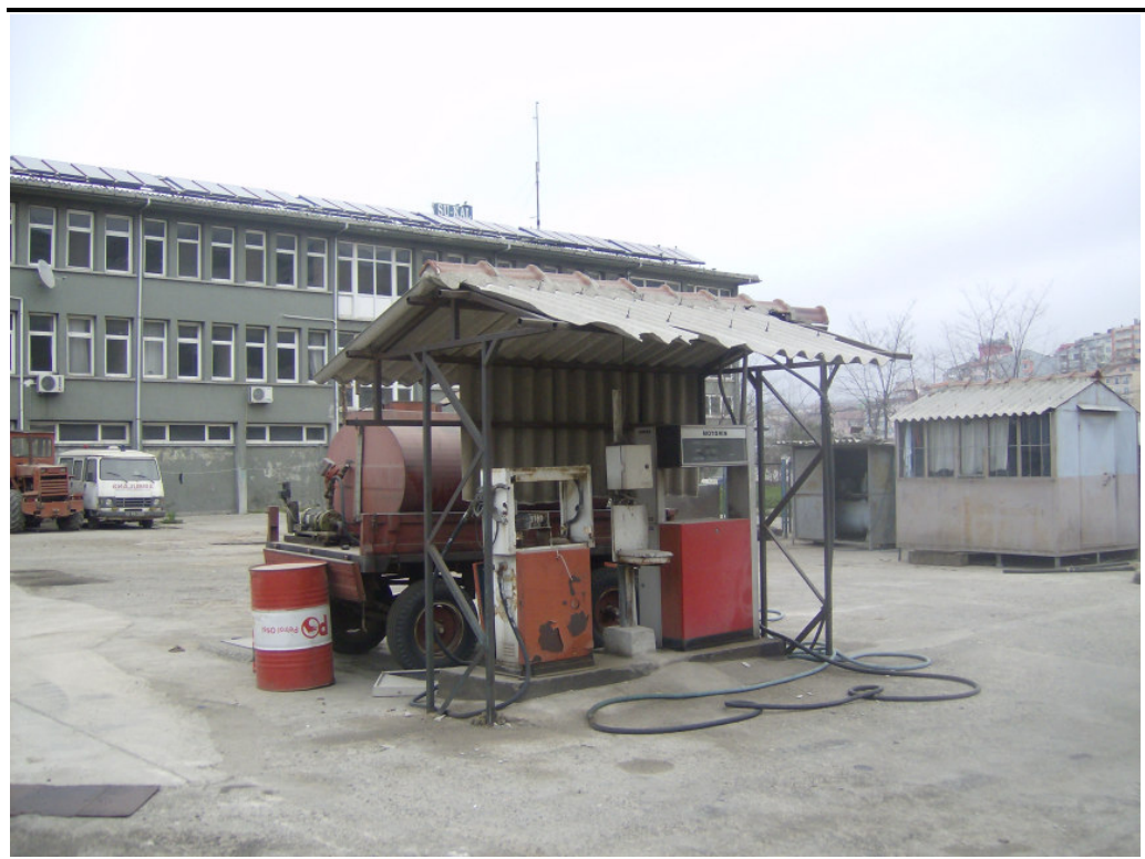
Box 1.6 Fuel Tank
