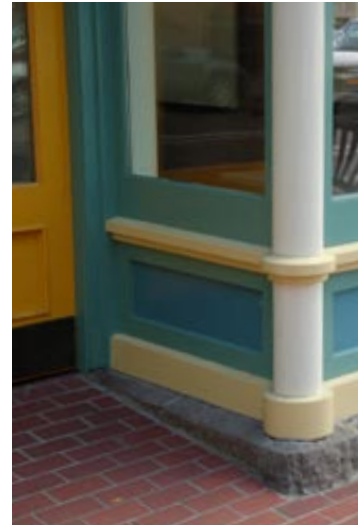
Wood window base on a durable stone base. The stone or concrete base provides extra protection from the water on the sidewalk.
