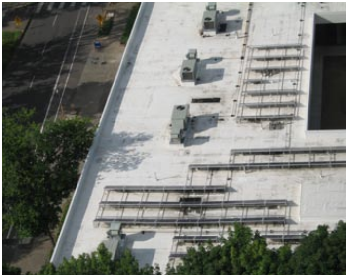
On site solar PV's are hidden from street view by this building's parapet (SW 1st Ave and Harrison St)
