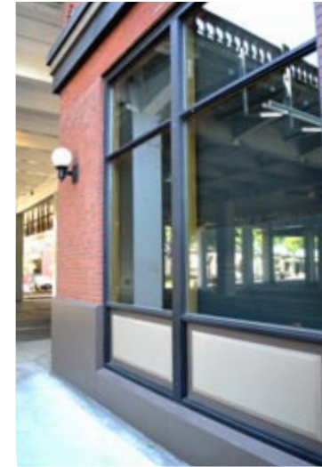
Contemporary storefront system example with aluminum-clad wood framed windows and integrated wood window base.
