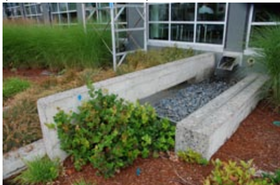
A roof drain integrates into the landscape as a flow-through planter. (SE Water Ave and Clay St)
