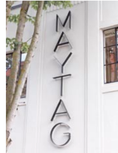
High contrasting colors are important to a successful pin-mounted letter sign.
