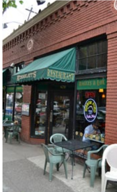
Awning example of maximizing transom day lighting while giving extra rain protection at the entry (NW 23rd and Irving St)
