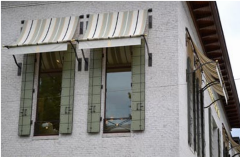
Operable awnings and shutters control how much sunlight enters the building (NW 23rd Ave and Flanders St)
