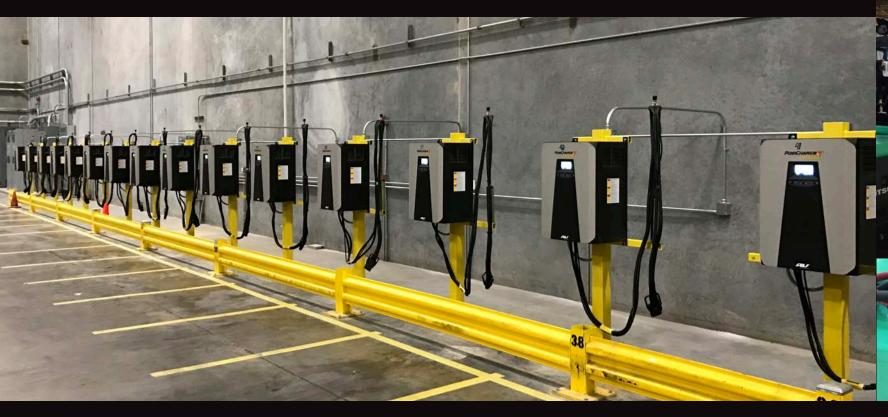
16 PROCORE 20KW UNITS WITH CHARGER STAND KIT & POGO STYLE CABLE MANAGEMENT
