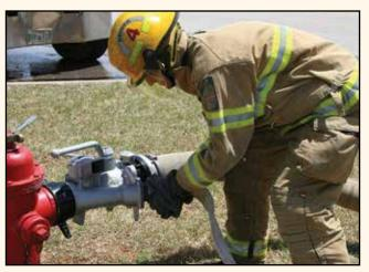
Step 5: Connect additional 2½- or 3-inch (65 or 77 mm) lines to gate valve and apparatus.
