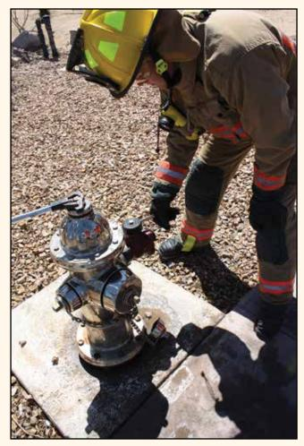
Step 3: Attach 2½-inch (65 mm) gate valves to hydrant.
