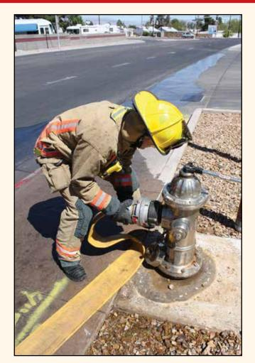
**Step 2:** Connect LDH to hydrant and lay hose to street, folding approx 3 feet (1 m) back onto itself (place two full counterclockwise twists in the hose if sexless couplings are not used).
