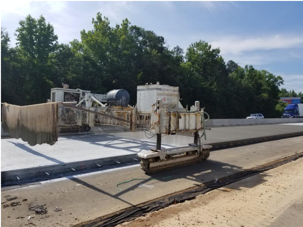
Figure 10: Application of curing compound.
