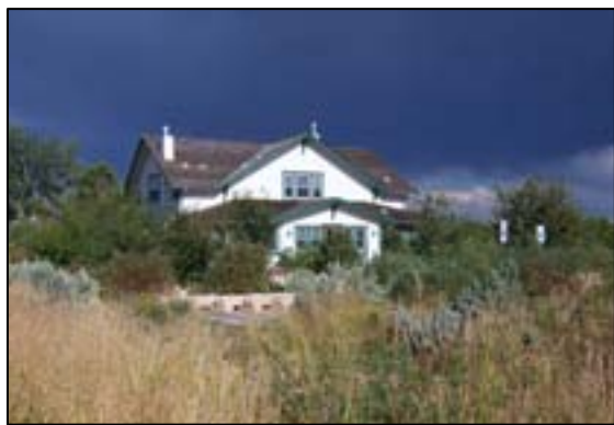
The historic Nix farmhouse was remodeled in 2002 and now serves as the main office of the Natural Areas Program.
