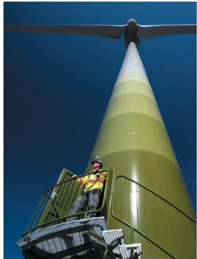
Wind turbine at Diavik Diamond Mine, NWT Courtesy of: Diavik Diamond Mine (2012) Inc.
