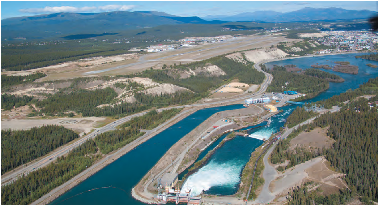
Whitehorse Rapids Generating Facility Courtesy of: Yukon Energy Corporation
