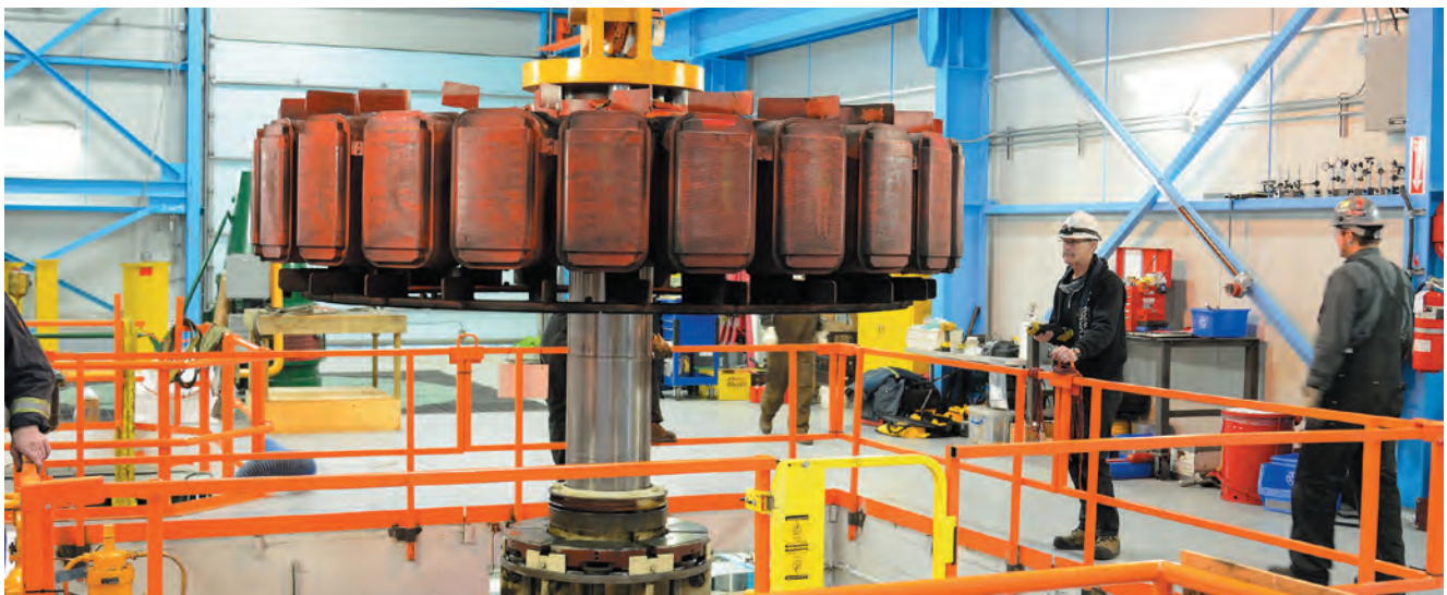
Repairs to hydro turbine, Yukon
