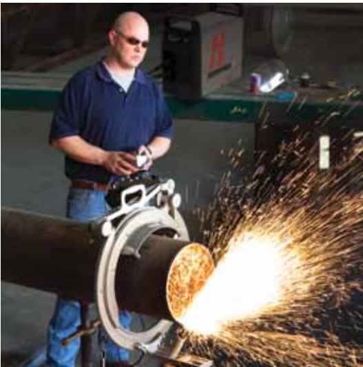
Pipe and bevel cutting
