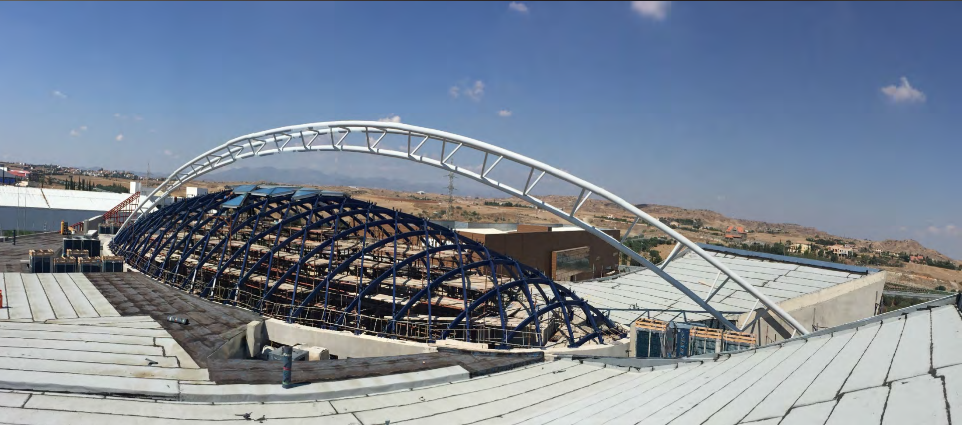
The above picture regards Project SEM in Cyprus – Fabrication, Transportation and Installation of Steel Roof and Arch
