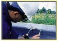
Figure 5: Zinc-Based Solder Technique
