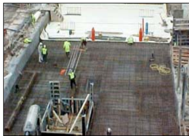
Figure 5.7 This prestigious commercial development incorporated the construction of a multi-storey office block with a link to a separate multi-storey car park. Yield Line Design was used for the flat slabs used in both of these blocks.
