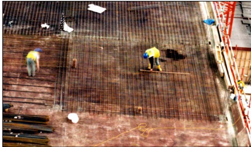
Figure 1.1 European Concrete Building Project at Cardington - 4 th floor during construction
