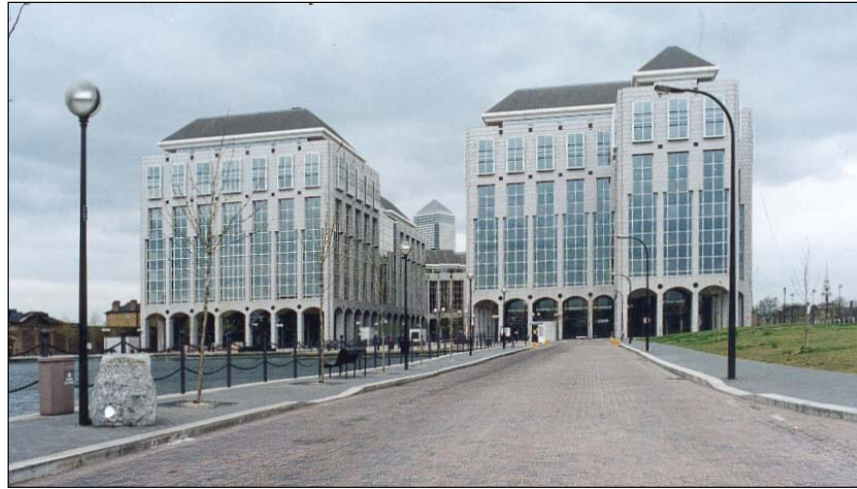
Figure 5.5 Four office blocks of 8 to 11 storeys make up this 1 million square feet development in London's Docklands. All the buildings consist of an in-situ concrete frame made up of a flat slab and columns.
