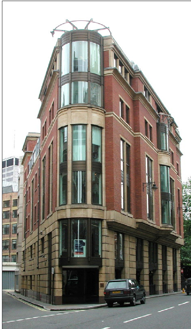
Figure 5.6 This £5 million project was located on a city centre triangular shaped site with two sides adjacent to busy London streets. The proposal called for a multi-storey office complex plus a two-level basement structure. Yield Line analysis was used extensively in the design of the triangular in-situ concrete flat slabs, together with the raft foundation.
