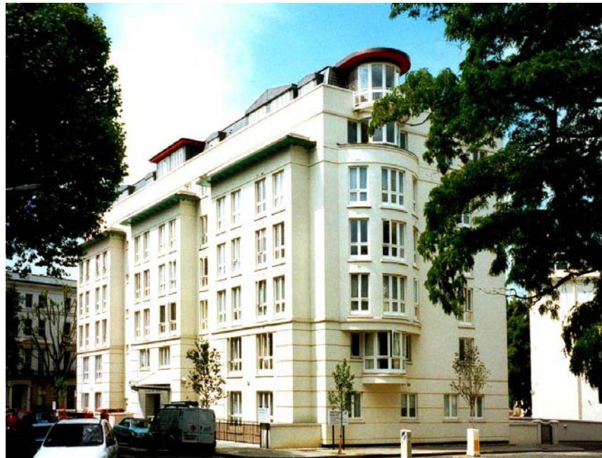
Figure 5.1 This is a multi-storey block of luxury flats with two levels of basement car parking.
