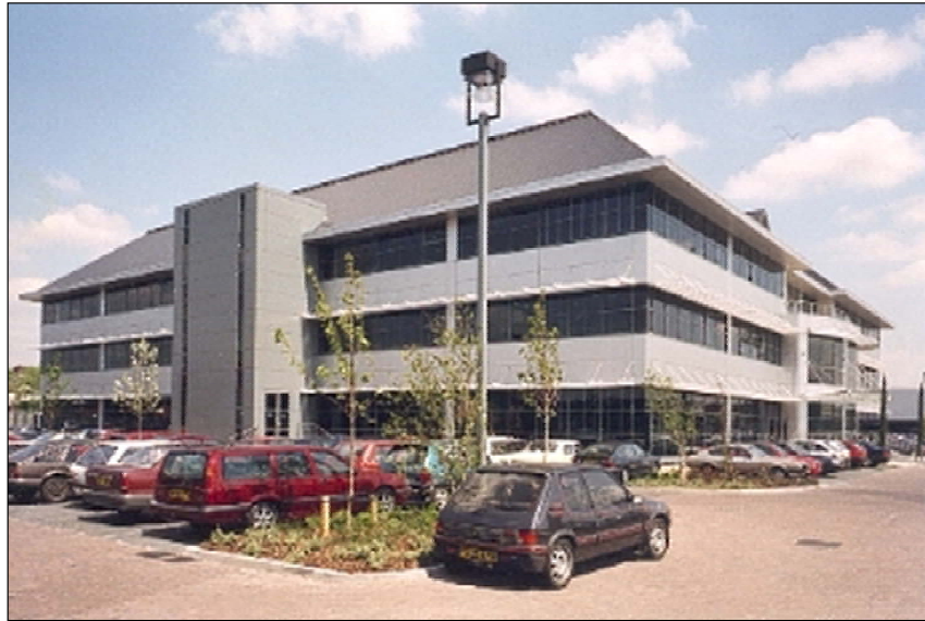
Figure 5.4 This project was constructed as the European Headquarters and central hub for Nokia. The building is a three-storey structure with two suspended reinforced concrete floors, covering a plan area of 54 by 54 metres. The columns are on a grid of approximately 9.5 m by 9.5 m supporting an r.c. waffle floor slab 450 mm deep overall.
