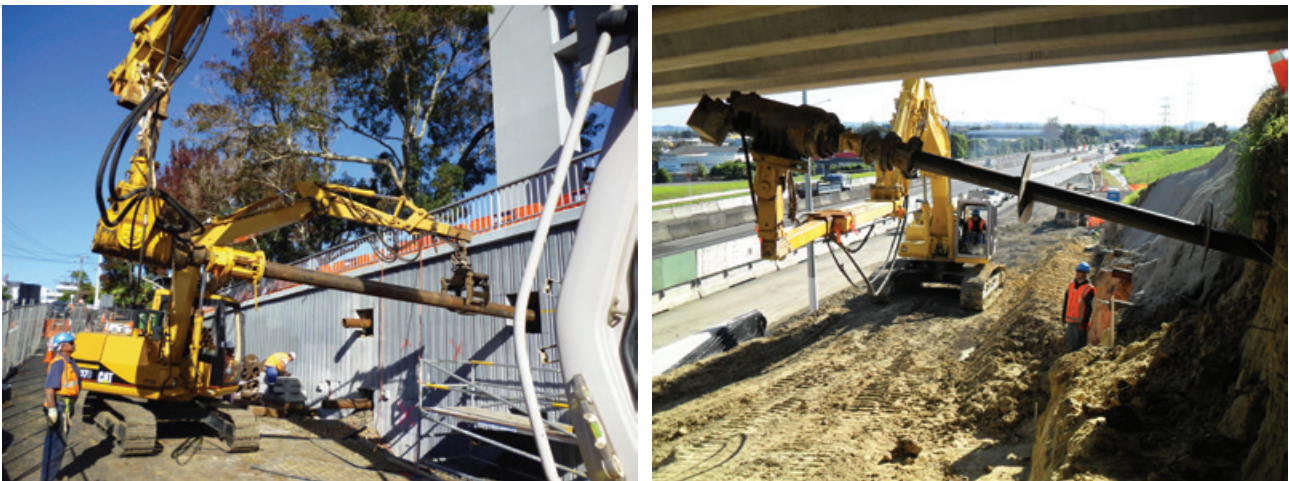
Figure 2.3: Screw Piles used for Anchoring
