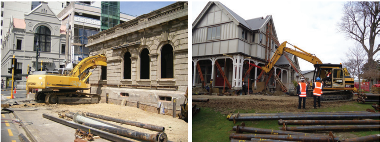
Figure 2.3: Screw Piles used for Anchoring
