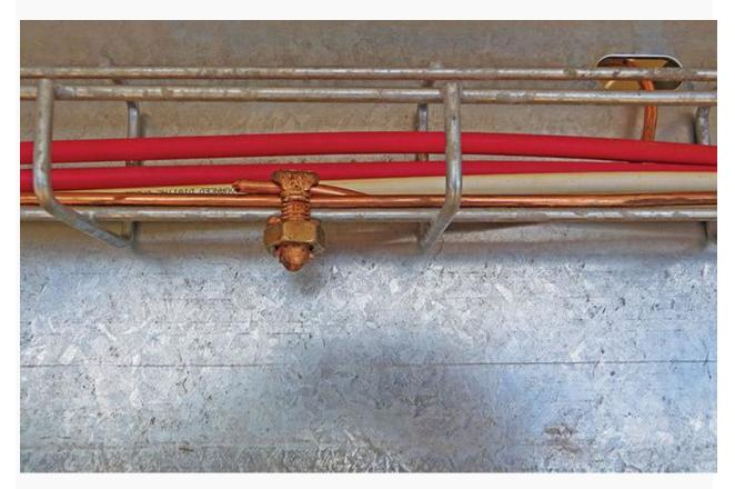
Grounding and bonding of cable trays (on photo: Ground wire connected to cable tray; photo credit: solarprofessional.com)
