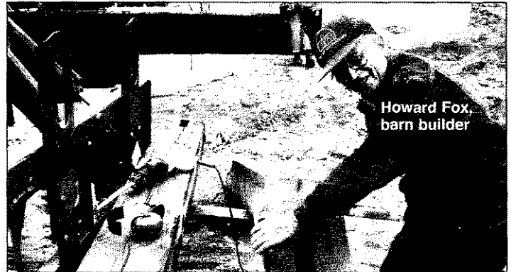
Nailing joist hangers for barn floor. Front to back: Mike Hansen, Dave Schoenholtz, Garrett Meiners, Dave S. Jr., and out of view, Erin Jones.
