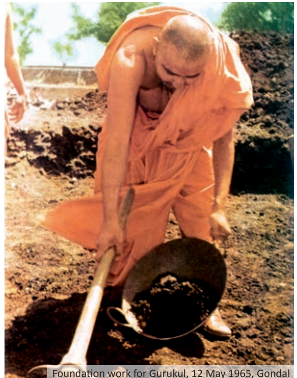
Foundation work for Gurukul, 12 May 1965, Gondal
