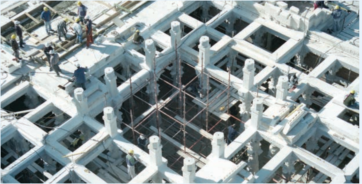
Construction of shikharbaddh mandir in London
