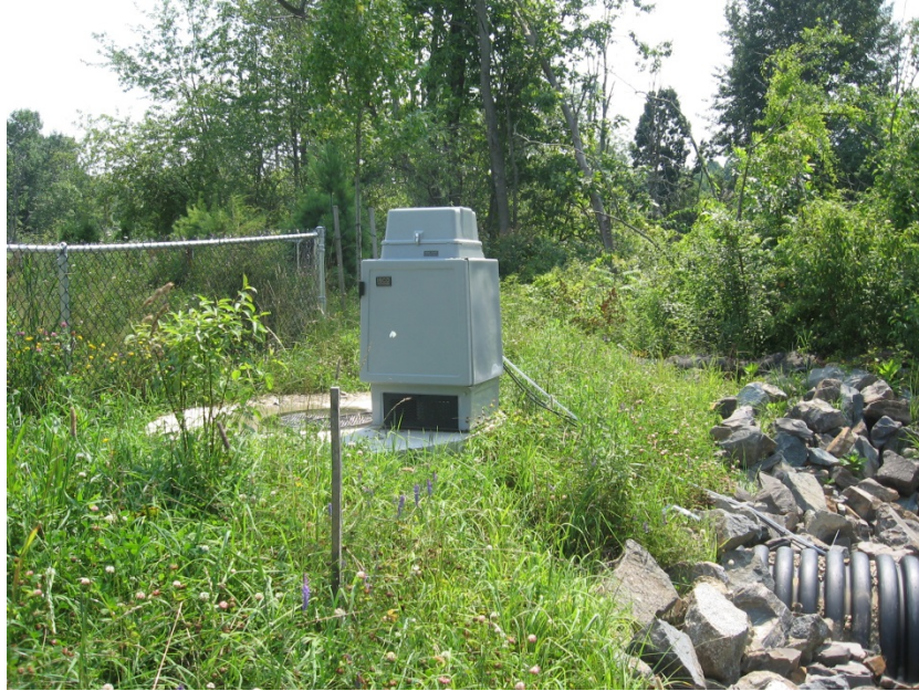
Figure 4: Teledyne ISCO 6712 Refrigerated Sampler installed at effluent location of subsurface gravel wetland.
