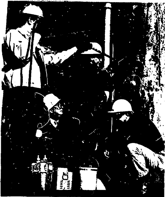
Graduate students take air pollution samples, from a coal-fired heating plant at West Virginia University, under normal test conditions. Another part of this class assignment was to measure the undesirable effects on a nearby building site.
