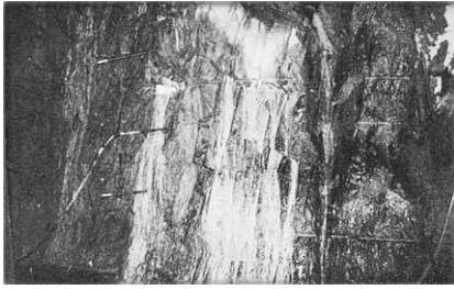
Figure 11.2 Acrylate grout appearing as limited backflow before sealing off
