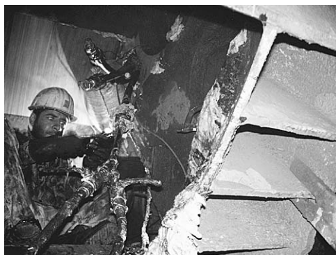
Figure 11.13 Injection of PU
