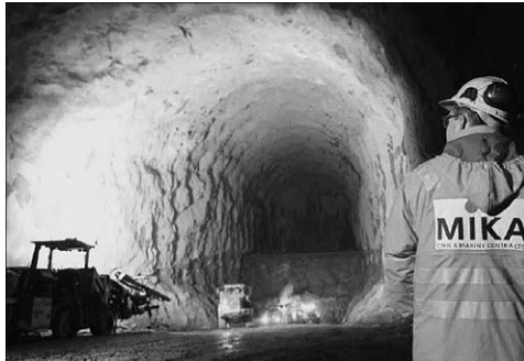
Figure 11.7 The propane storage cavern at Mongstad, Norway
