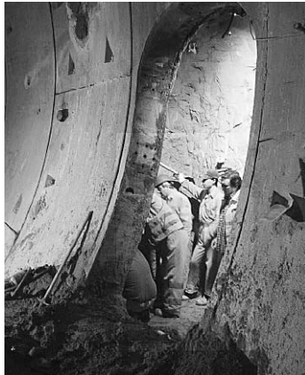
Figure 11.11 Cross passage excavation after injection
