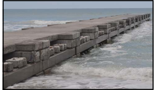
MARINE STRUCTURE FOR EROSION CONTROL
