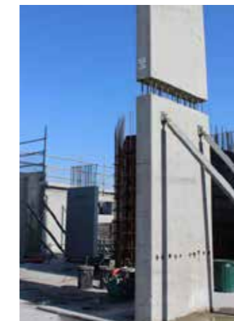
Double Height Column With minimum prepping
