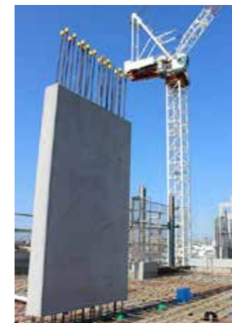
Double Height Column With upper part pre-installed
